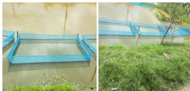
Fig 1: Installation of hapa
