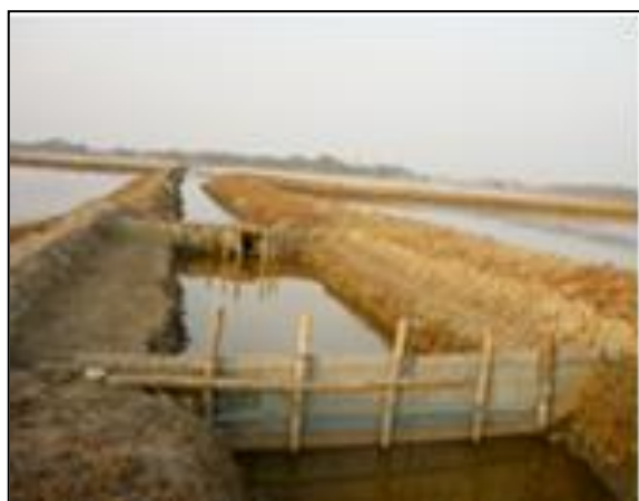
Plate 1: Fishpass (allowing fish movement between Gher to Gher)
