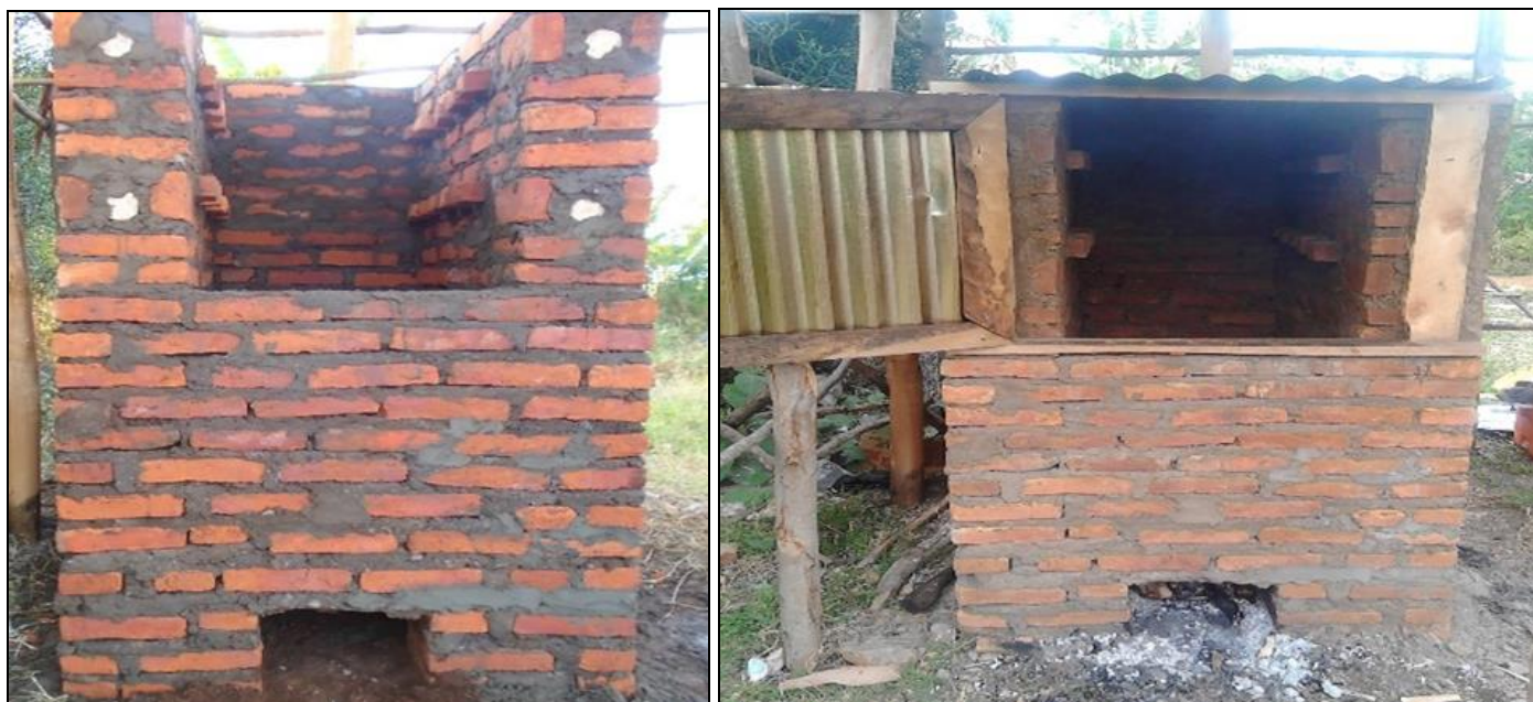
Fig 1: Front view of adopted simple Altona oven
