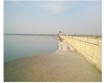
WALL OF THE DAM
