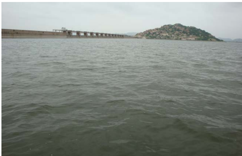
Fig 3: Inner view of Koilsagar reservoir
