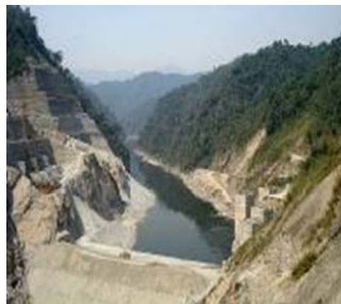
Dam site of R. Subansiri during construction
